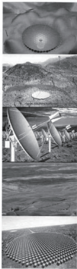
Options for the stations of the SKA, from the top: A set of large (>300m) spherical reflectors; A large (>200m) reflector with the receiver supported by an antenna; An array of small (<10m) parabolic dishes; A fixed element (electronically phased) array. An array of spherical (>10m) refracting lenses.
